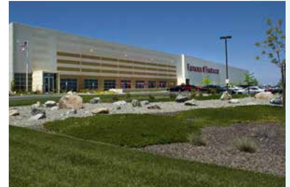
Low profile landscaping at the Famous Footwear distribution center at Tejon Ranch Commerce Center is well maintained and provides good visibility to the building yet creates a buffer to the parking lot.
