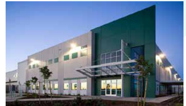
A variety of materials and color can create visual interest along a building.
